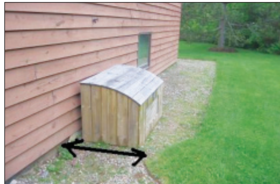
Not Recommended (Wooden, unlocked, too close to building)
