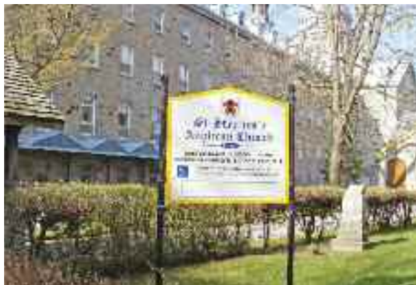
AFTER MANY MONTHS of talking and planning, a new sign is in place at St Stephen's Lachine, which really took to heart a suggestion made by the 2010 report to the Diocese by consultant Myrlene Boken report that the church be more visible in the community. "Last year we painted our new restored window frames bright yellow, then this year we had the border on our new sign match them. In fact, following a recent overheard comment, we are thinking about calling ourselves the 'Sunshine Church,'" says parishioner Mary Pickup.
