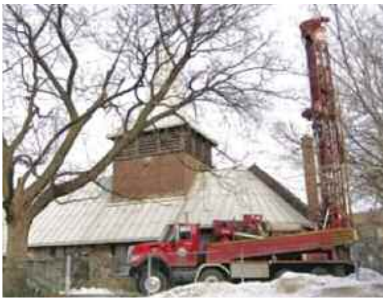
DRILL RIG near chapel.
