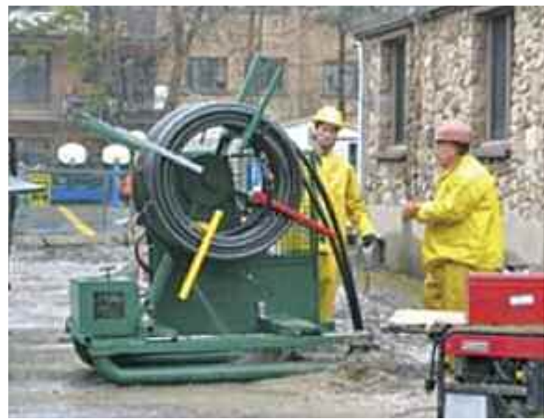
INSERTING CABLES into wells.
