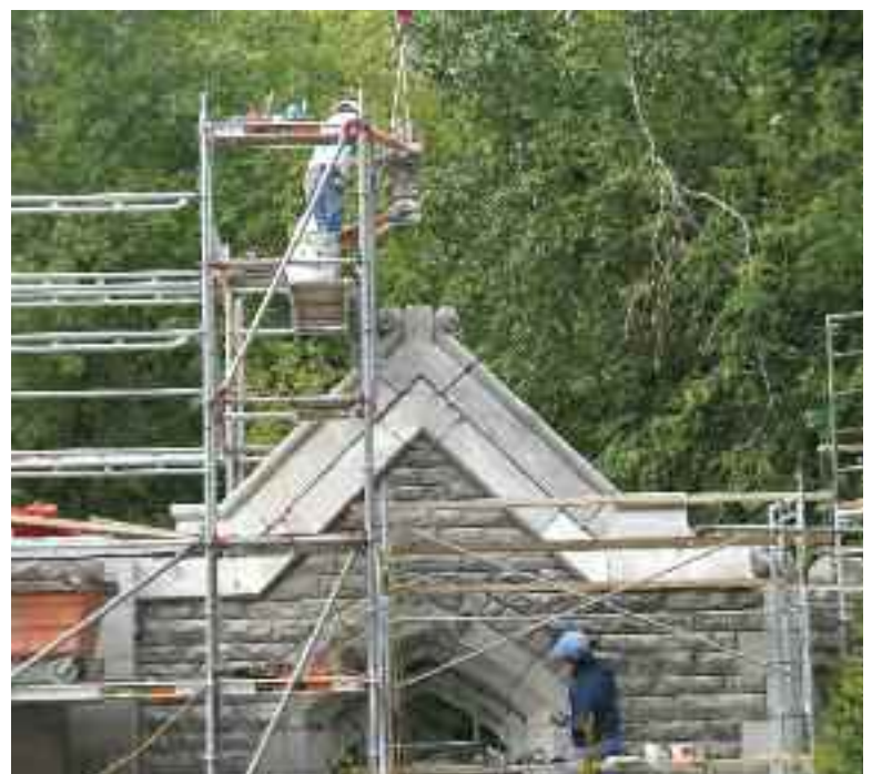
The gate restoration project in progress, September 2014 (Photo: Mark Gallop)
