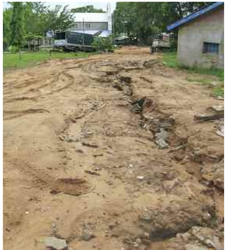
ONLY ACCESS to the Cathedral compound, badly eroded during construction of the water supply system and not repaired.
