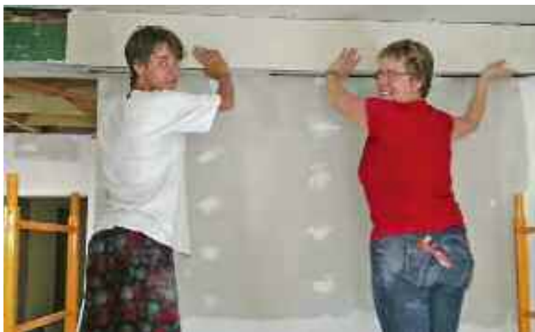
VOLUNTEERS Mike Biever of St Stephens Westmount and Fiona Crossling of St. Peter's TMR instal drywall.
